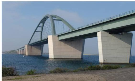
**Fig. 2:** Fehmarnsund network arch bridge
