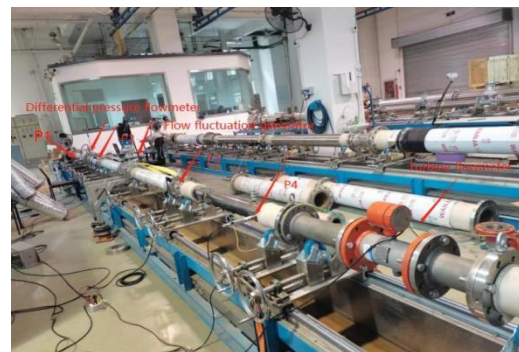
Figure 9: Pipeline installation site map.
