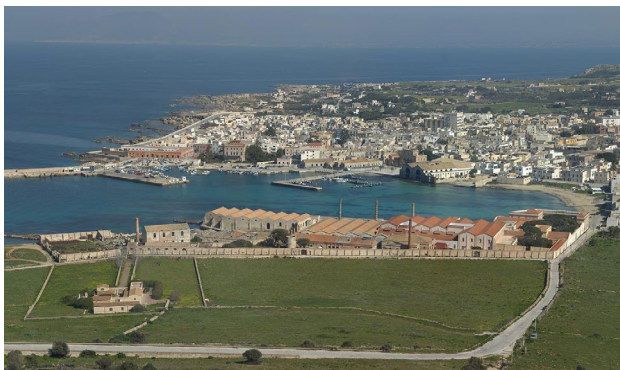
Fig. 1. General view of the former Tuna Factory "Florio" in Favignana | © D. Pavone, CNR ISPC.
