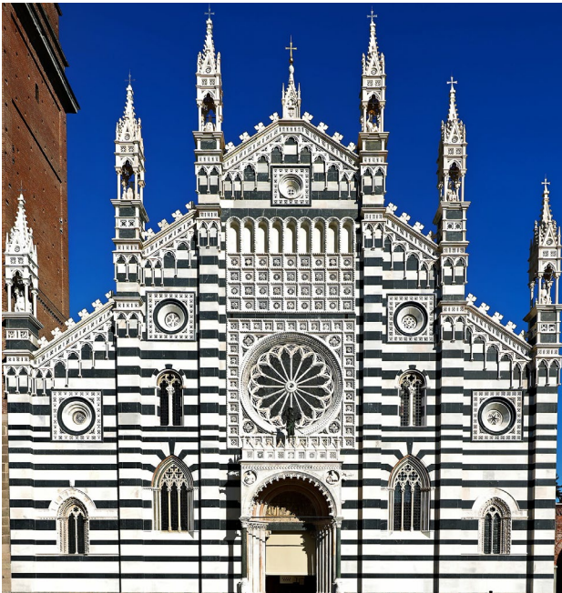
Fig. 1. Photograph of the façade of the Monza cathedral (Monza, Italy).
