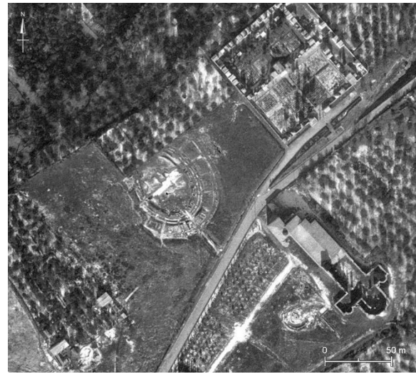
Figure 2. Excavated structures of the amphitheater area in a historical aerial photo taken by S.A.F. ( Società AeroFotografica ) in 1964.
