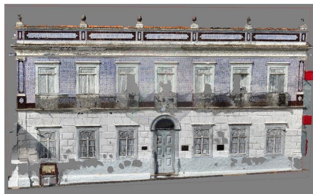
Fig. 6. Photogrammetry software arranging images generate dense cloud and texture data of the MRCI main façade, MRCI/MP/USP.
