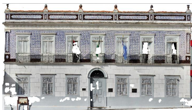
Fig. 7. Photogrammetry orthoimage of the main façade of the MRCI, MRCI/MP/USP.
