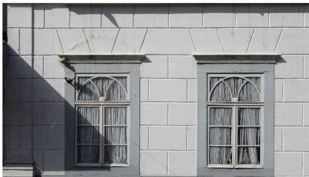
Fig. 4. Drone photography of the MRCI main façade, MRCI/MP/USP.
