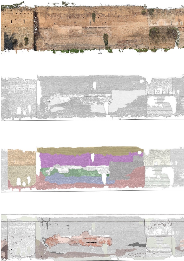
Fig. 1. Documentation and representation of the Aurelian Walls of Rome. Towers L39-40.
