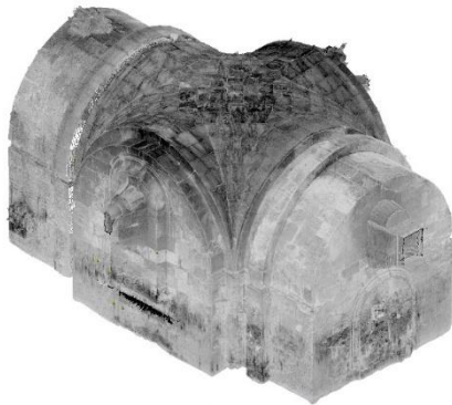
Fig. 8 – Point cloud of the intrados of the lower environment (MC processing).
